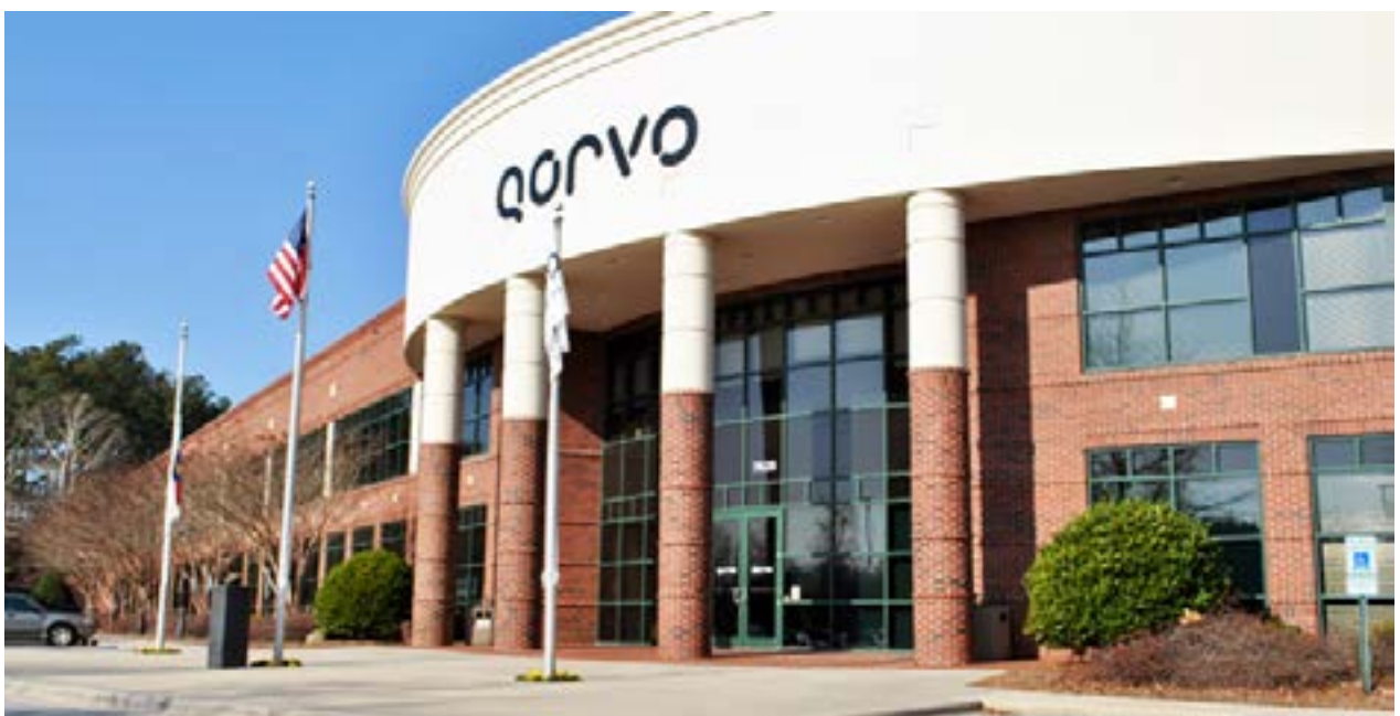
Qorvo's headquarters in Greensboro, NC is also a design, sales, support center and GaAs/GaN manufacturing facility.
